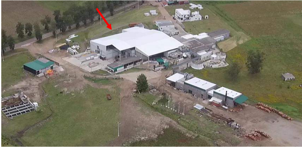
New building at Clay slaughterhouse
