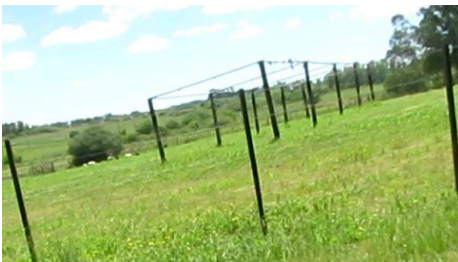
Broken shelter without roof at "acopio"
